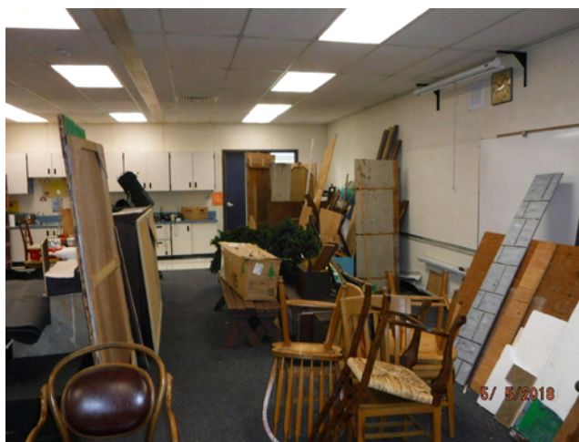
17 Classroom #7 Interior (c).JPG 05/05/2018
